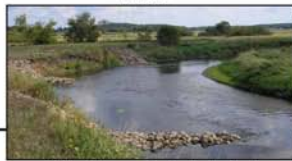
After Stream Barbs Installed
