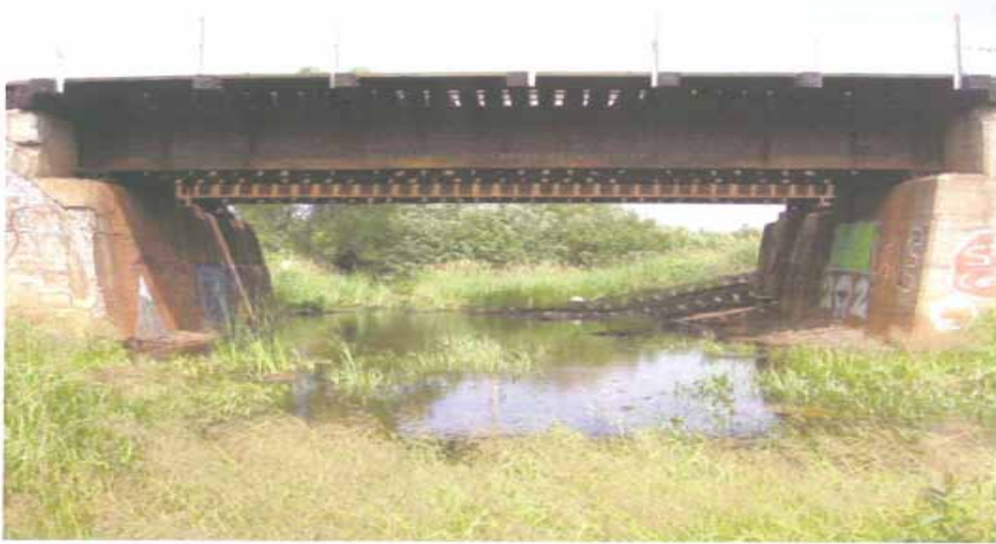
Upstream Face Looking Northeast
